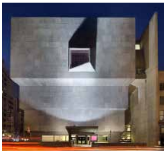
5. Third building of the Whitney Museum by Madison Avenue, now the Met Breuer Museum, Metropolitan Museum of Art, https://www.inexhibit.com/wp-content/uploads/2016/03/The-Met-Breuer-facade-Madison-Avenue.jpg
